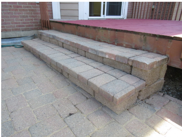
Block stairs to porch - Could come loose
