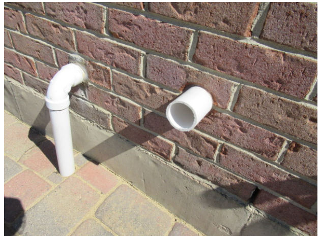
Open pvc pipe to the left of back porch - Most likely for the sump pump
