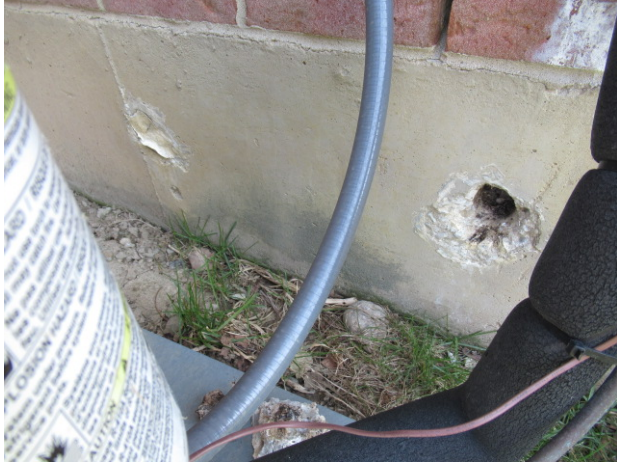
Holes from previous air conditioner in foundation
