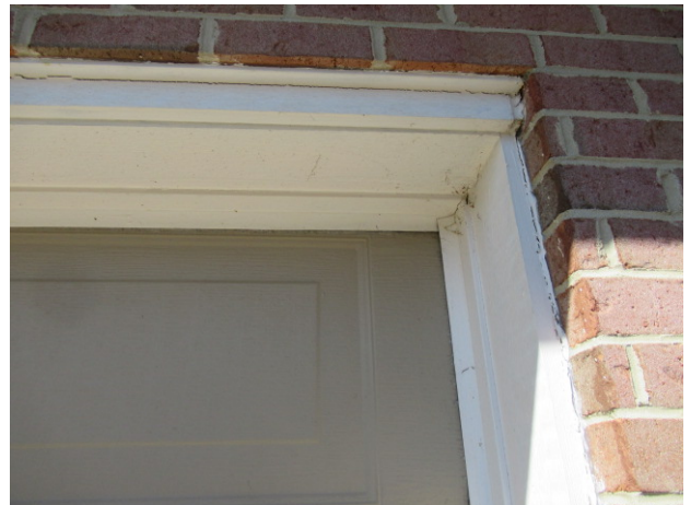
Caulk is in poor condition around garage door trim
