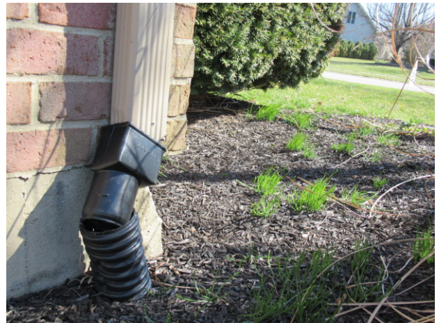
Down spout disconnected from drain pipe
