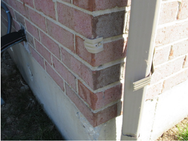
Broken down spout - Sharp edges
