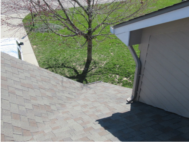
Down spout draining onto roof
