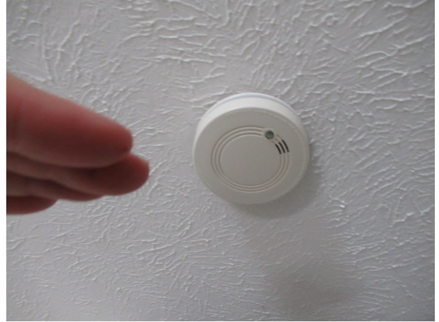
Possibly defective smoke alarm in basement - beeped very quietly when tested
