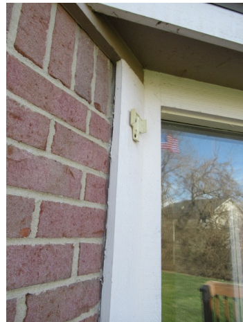
Caulk in poor condition on trim - to the left of window over the porch
