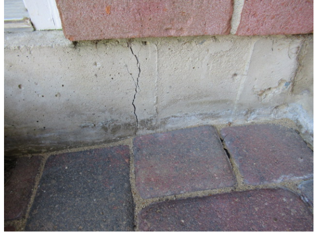
Example of minor settling cracks in foundation
