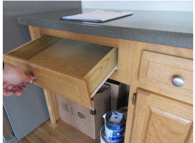
Broken drawer sliders on desk in kitchen
