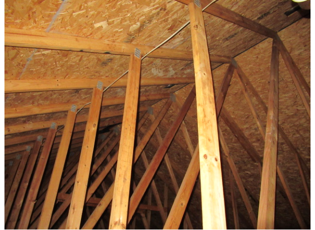
OSB sheathing in excellent condition
