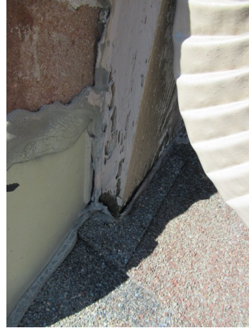
Paint and caulking damaged behind down spout on roof above garage
