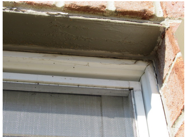
Multiple windows need to be recaulked around trim
