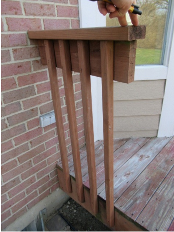
Improperly secured rail on back porch
