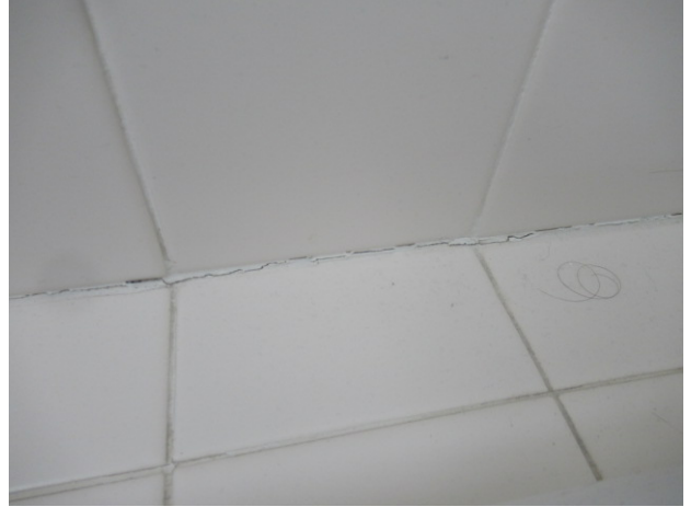
Caulk in poor condition around Jacuzzi tub
