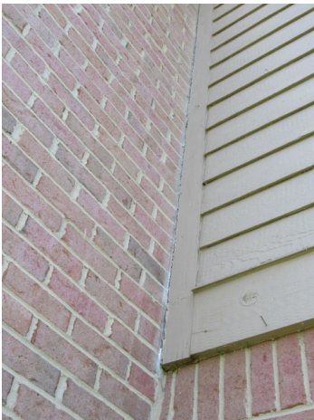
Caulk between chimney and siding is in poor condition
