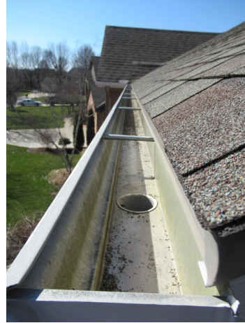
Gutters are clean other than some granules - typical amount for a mid-life roof
