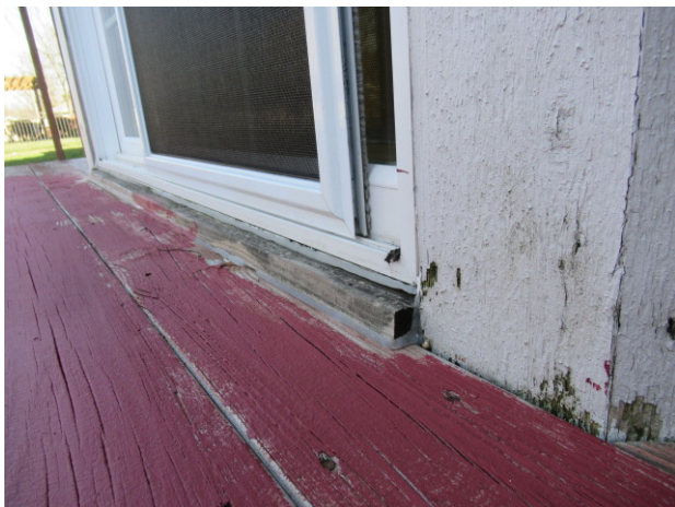
Trim and threshold paint are in poor condition - Wood beginning to show signs of rot
