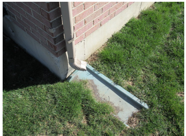
Trough is not placed correctly
