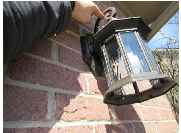
Light fixture is loose - right side of garage
