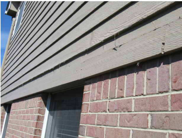
Paint on drip edge is in poor condition
