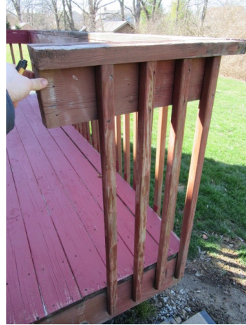
Improperly secured rail on back porch
