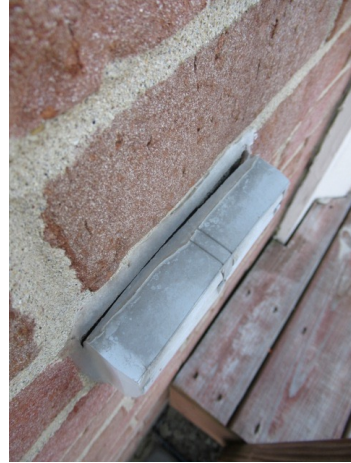
Outlet just off back porch - Missing caulk
