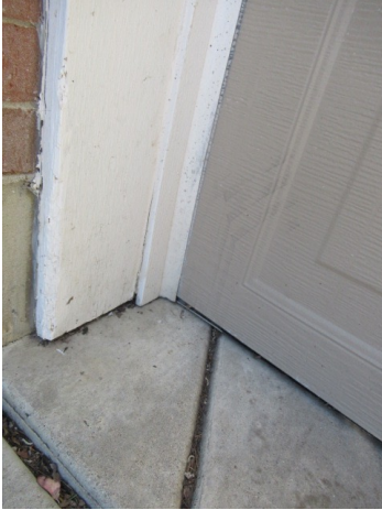
Paint in poor condition at base of garage door trim
