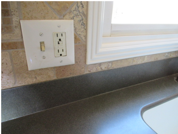
Broken reset switch - still functions GFCI above desk in kitchen is not functioning (No pic)
