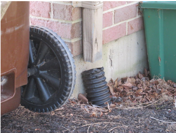
Down spout disconnected from drainage pipe
