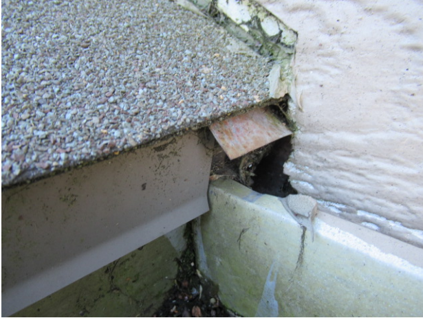
Loose flashing above gutter - Above back door
