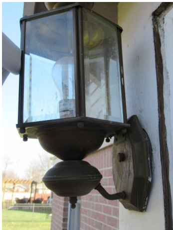
Light fixture is loose - back porch
