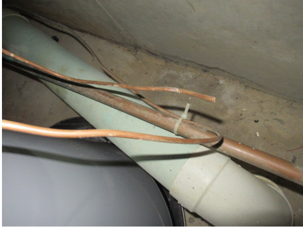
Zip tie used to attach ground to water pipe
