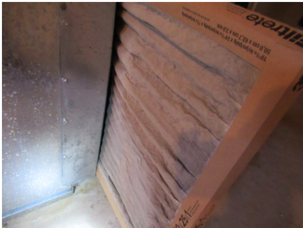
Dirty filter, needs replaced
