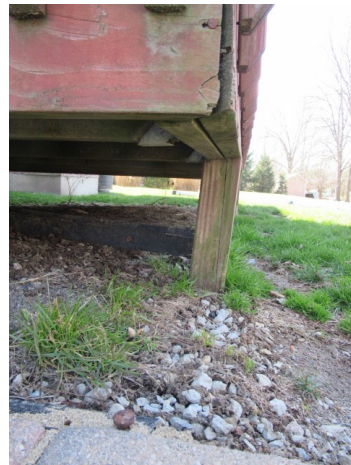
Crooked deck supports
