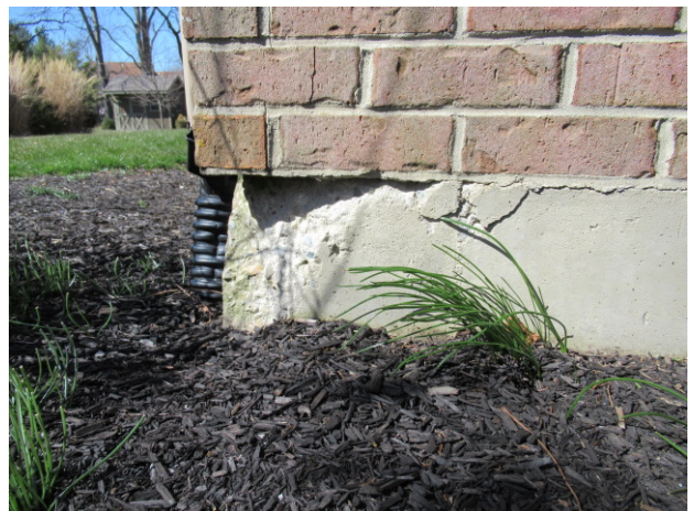
Corner of foundation damage - front left of home
