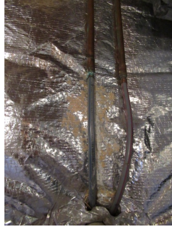
Evidence of water leak from hose - to the left of furnace
