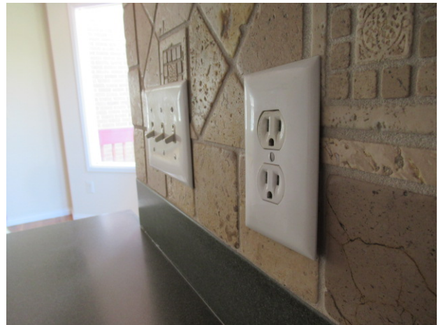
Outlets/plates on left and right side of counter are loose on bottom
