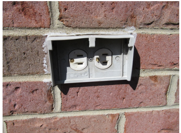
Missing outlet cover - Front of house
