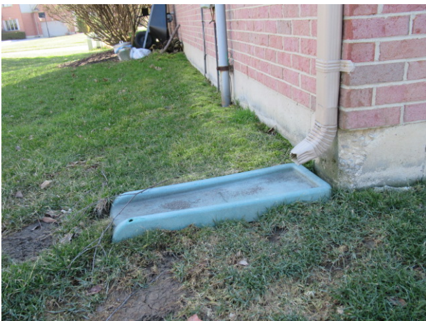
Down Spout trough is leaning slightly towards foundation
