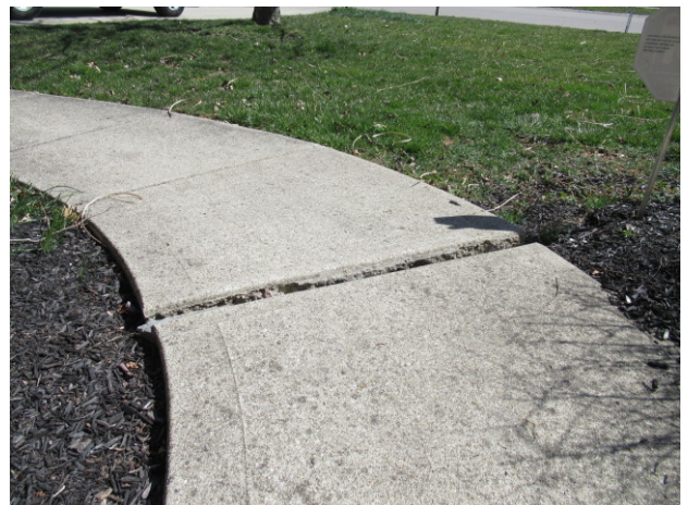
Tripping hazard near the front step
