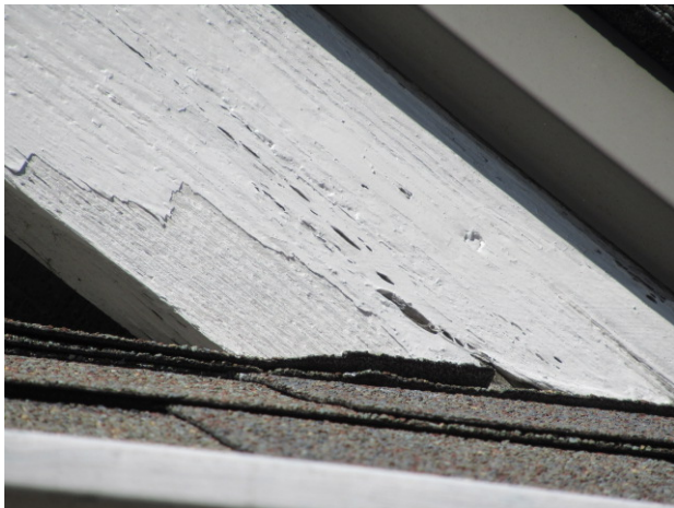
Paint chipping on fascia above garage - Front of house
