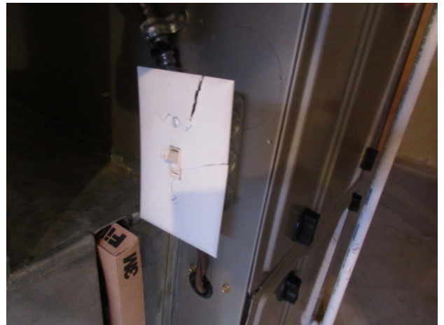
Broken plate on furnace shutoff switch
