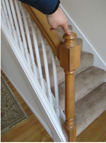
Improperly secured rail on stairs
