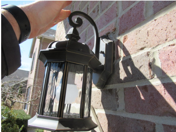
Light fixture is loose - left side of garage
