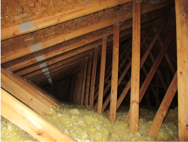
Sufficient insulation
