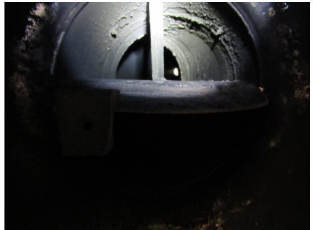
Light debris in chimney - damper does not fully close
